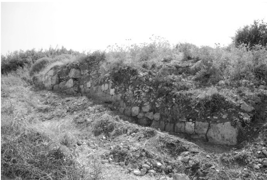
FIGURE 2.10 A section of the external fortifications of Antioch, possibly dating to the early Roman period
